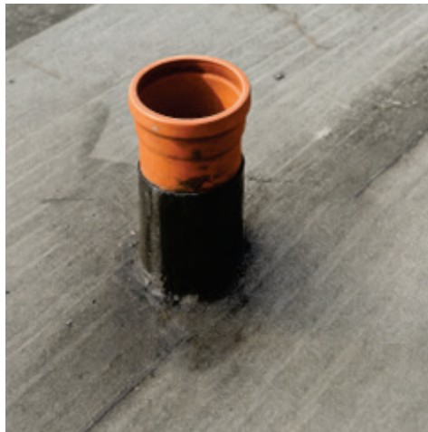
Figure 3 Raising of bitumen on the pipe feedthrough
